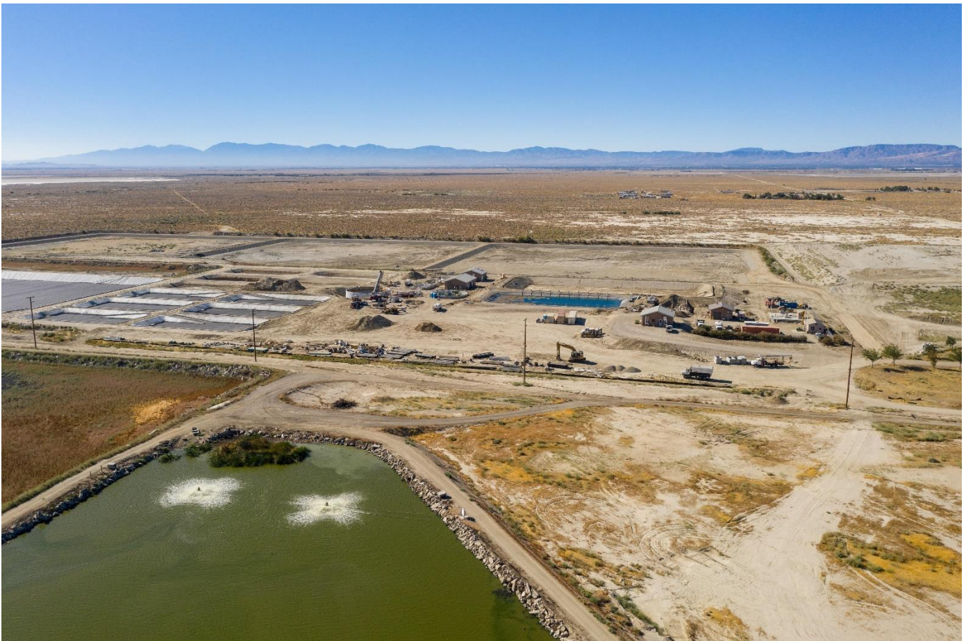
Figure 1-2: Ongoing upgrades to District's WWTP, Aug. 2020
