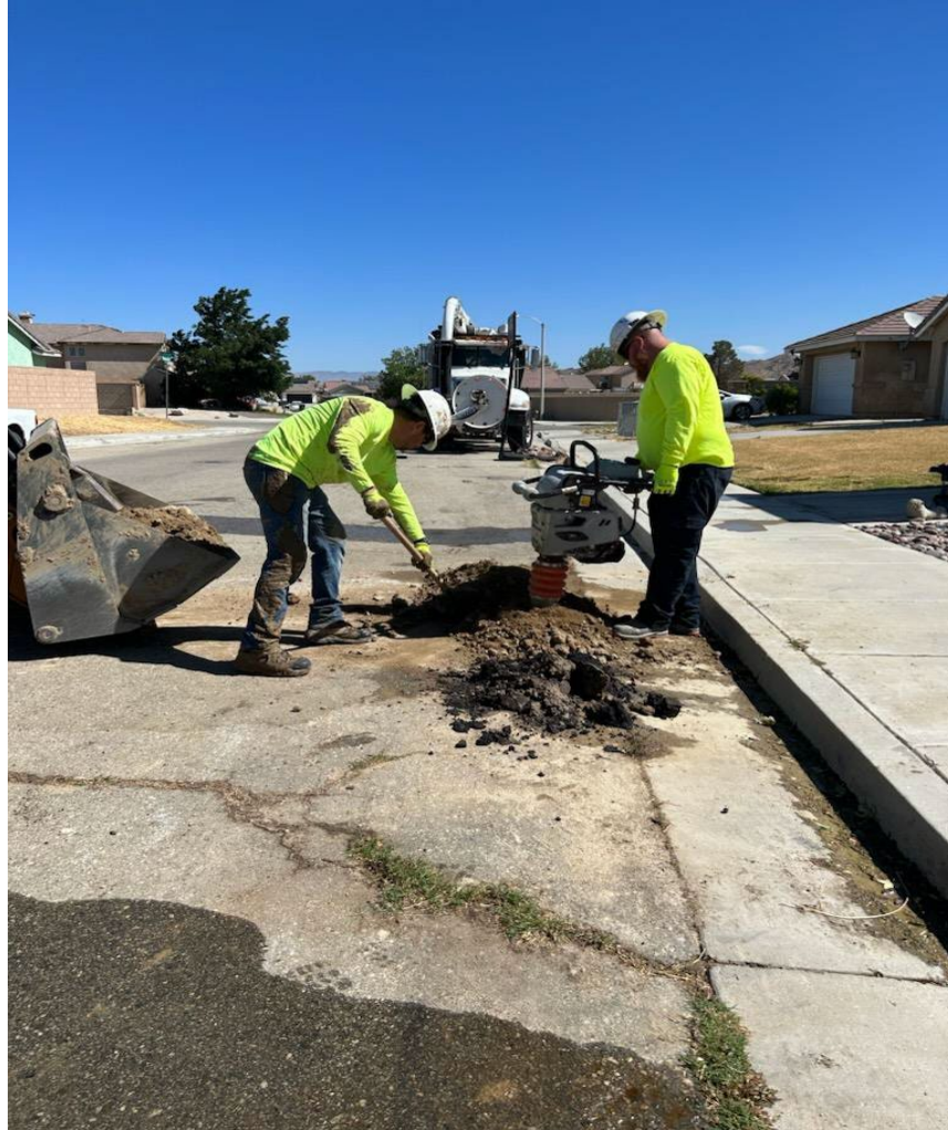
( Operators Dago Herrera and Tim Seufert fixing a leak )
