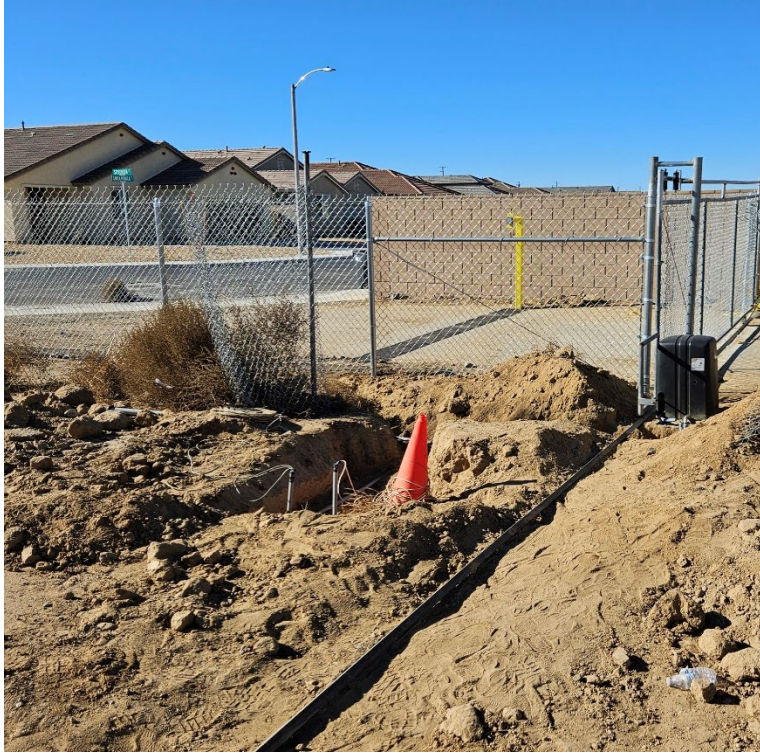
New rear gate entrance installation
