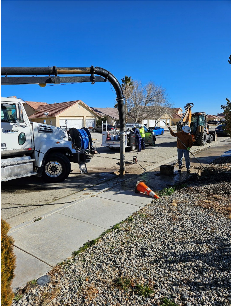
Water crew repairing a leak on Cold Creek ave
