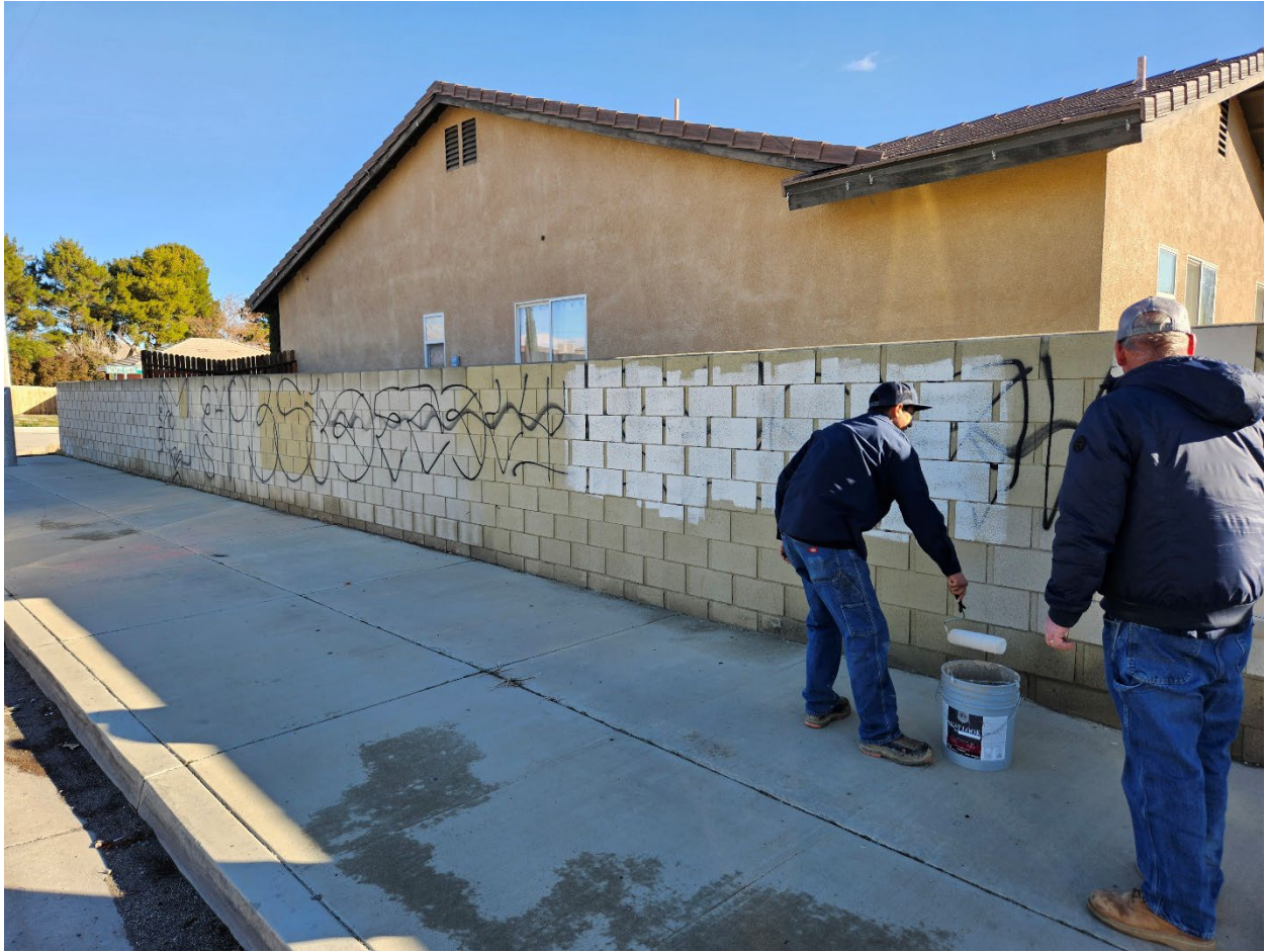
Staff removing graffiti on 15th st west.
