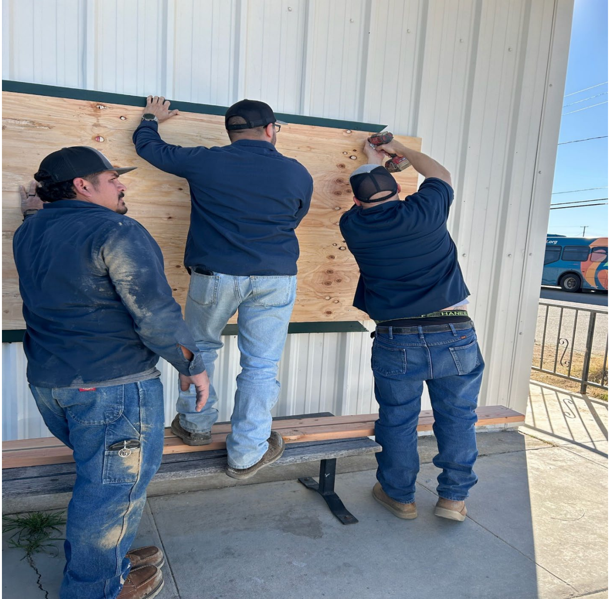
Staff boarding up broken windows on 20th st building
