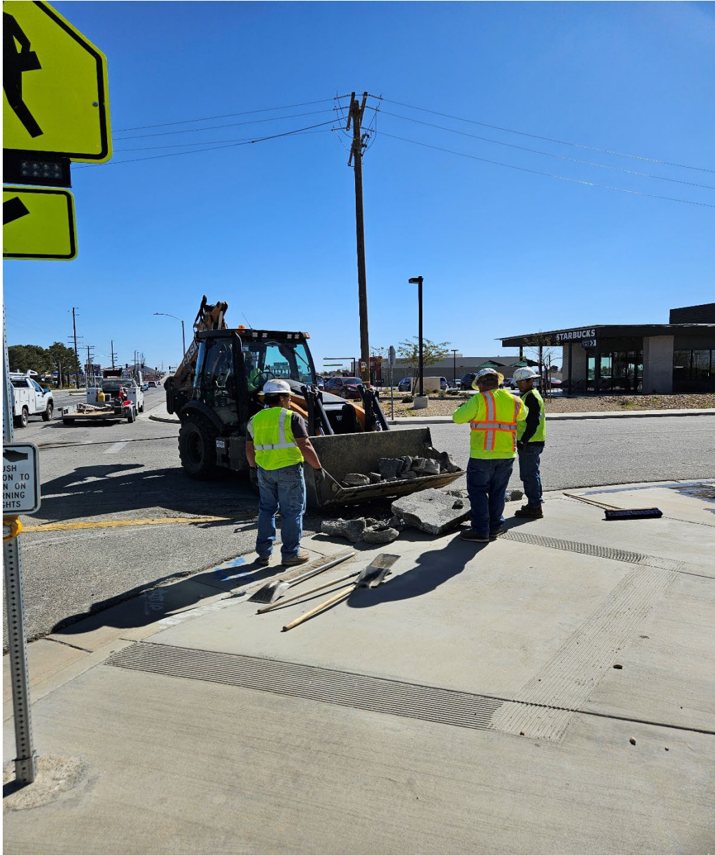
Public Works staff removing concrete debris from lowered water valve cluster.
