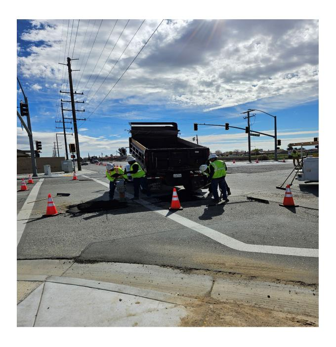
Staff covering lowered facilities with cold patch asphalt
