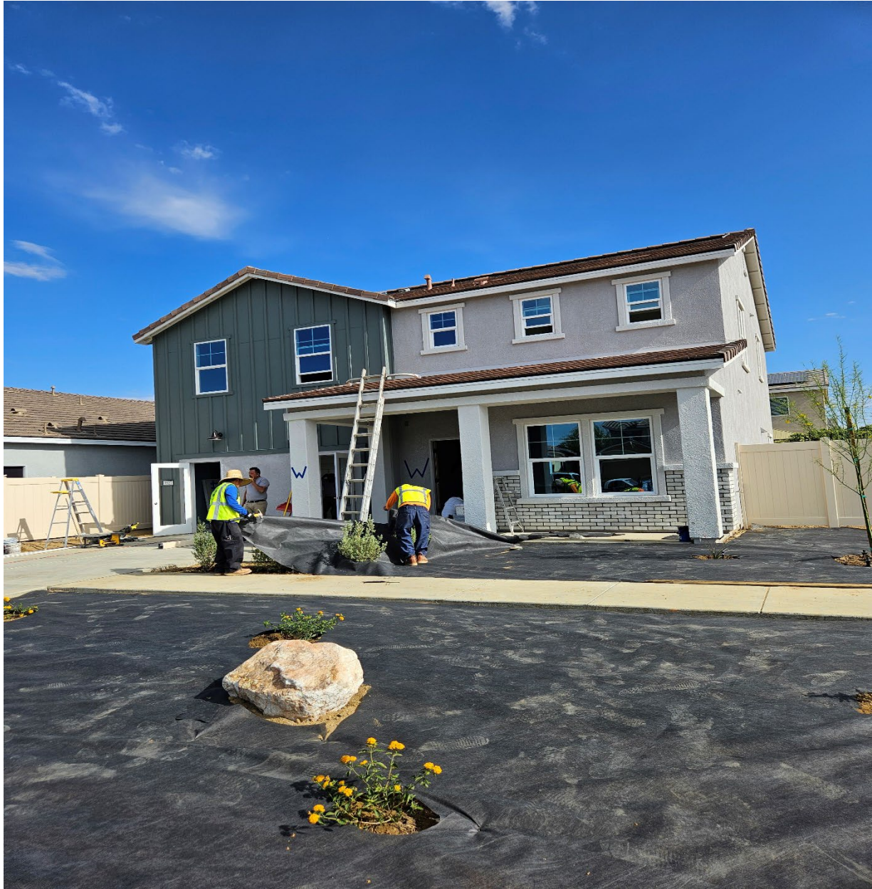
K. Hovanian model home nearing completion
