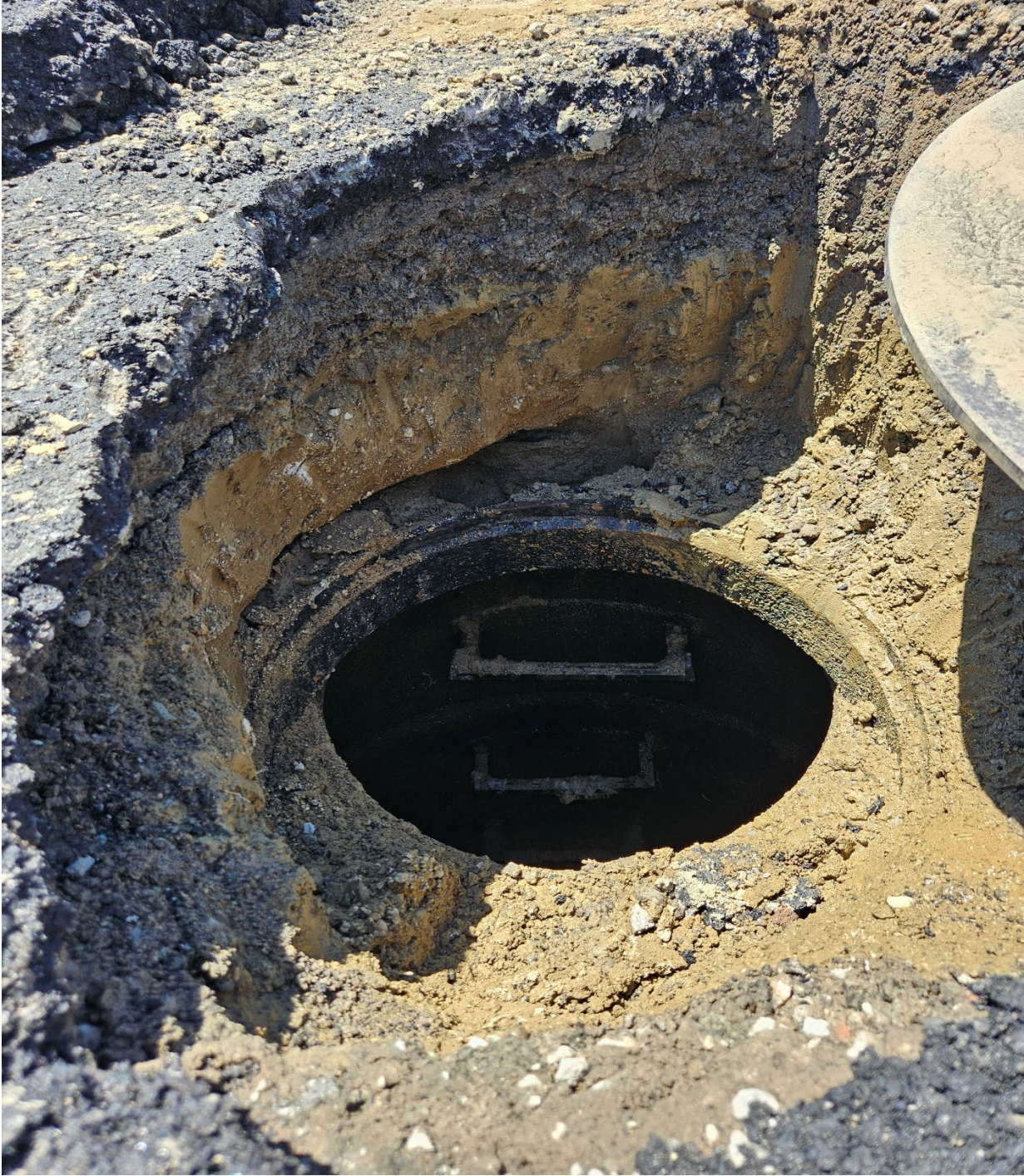
Covered manhole located and exposed
