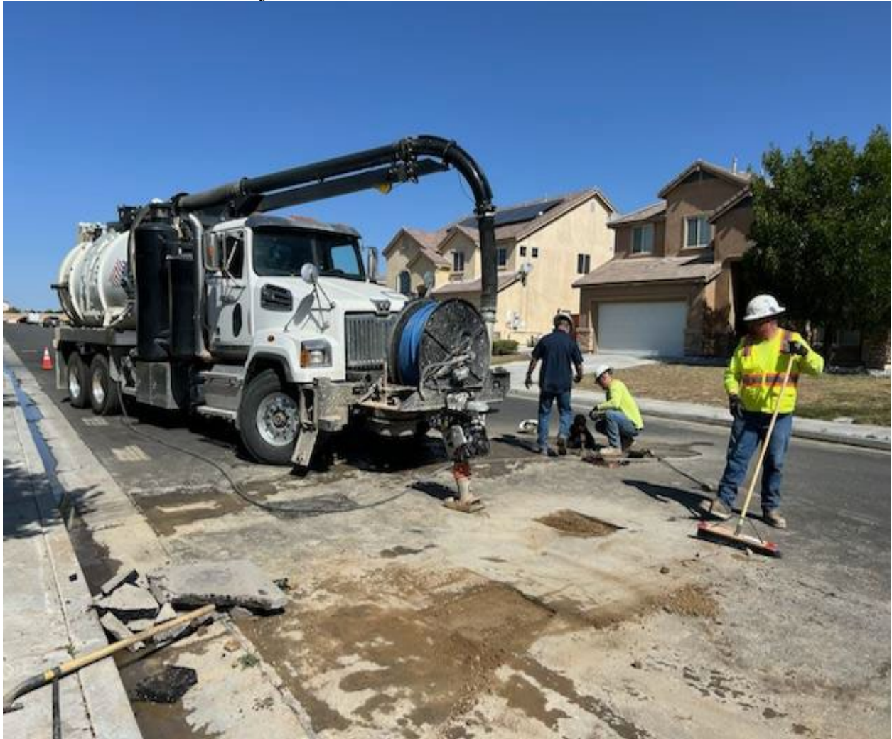
Leak repair by Public Works Dept
