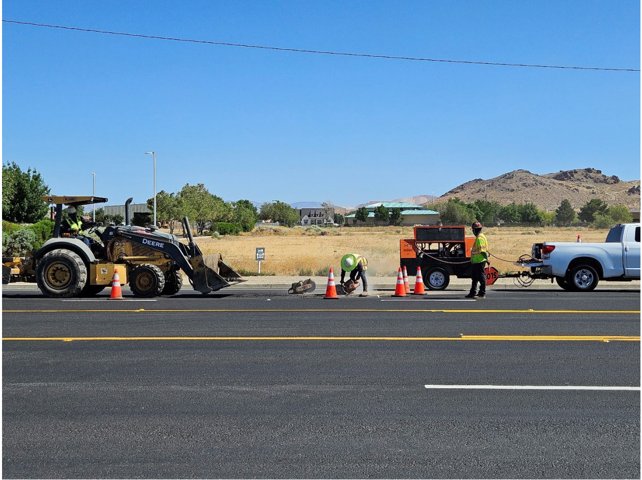
Bowman Asphalt Construction raising our sewer manholes after paving.
