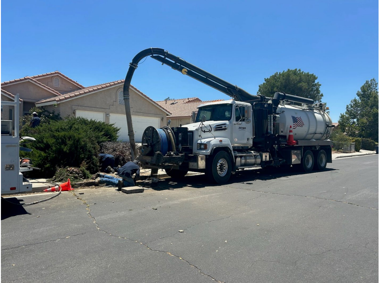
Public Works staff repairing leak with vacuum truck.
