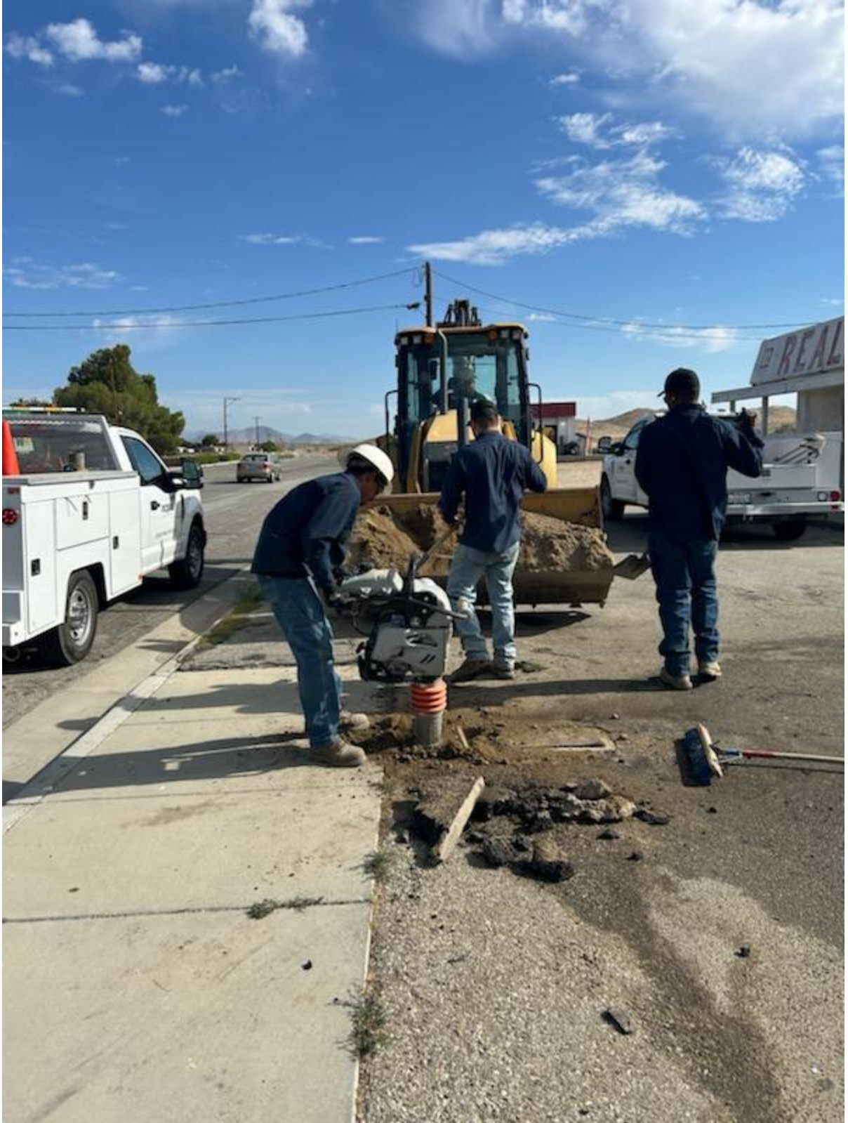
Public Works Staff repairing a water leak
