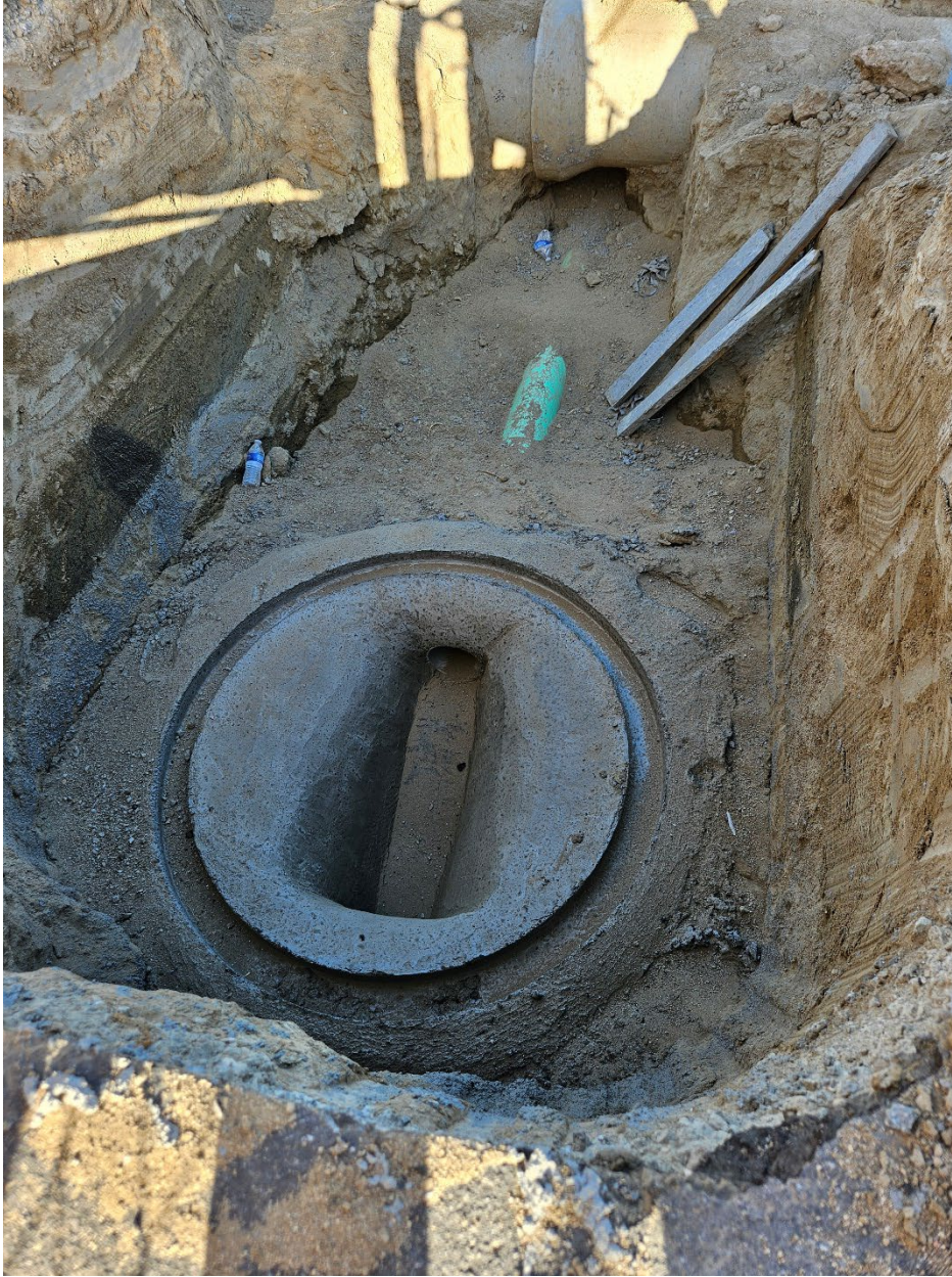
Sewer manhole being built for new track on Poplar
