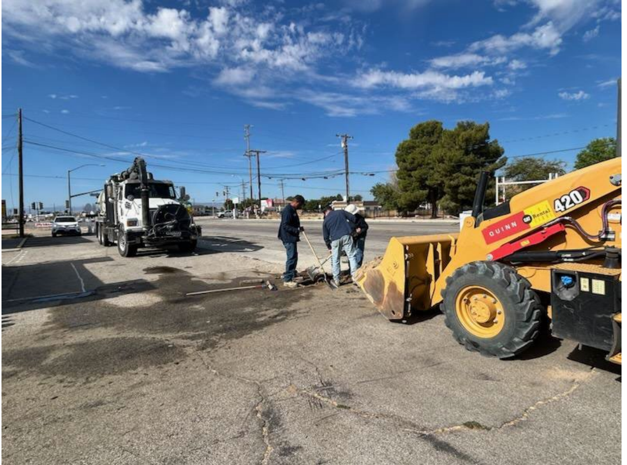
Public Works Staff repairing a water leak
