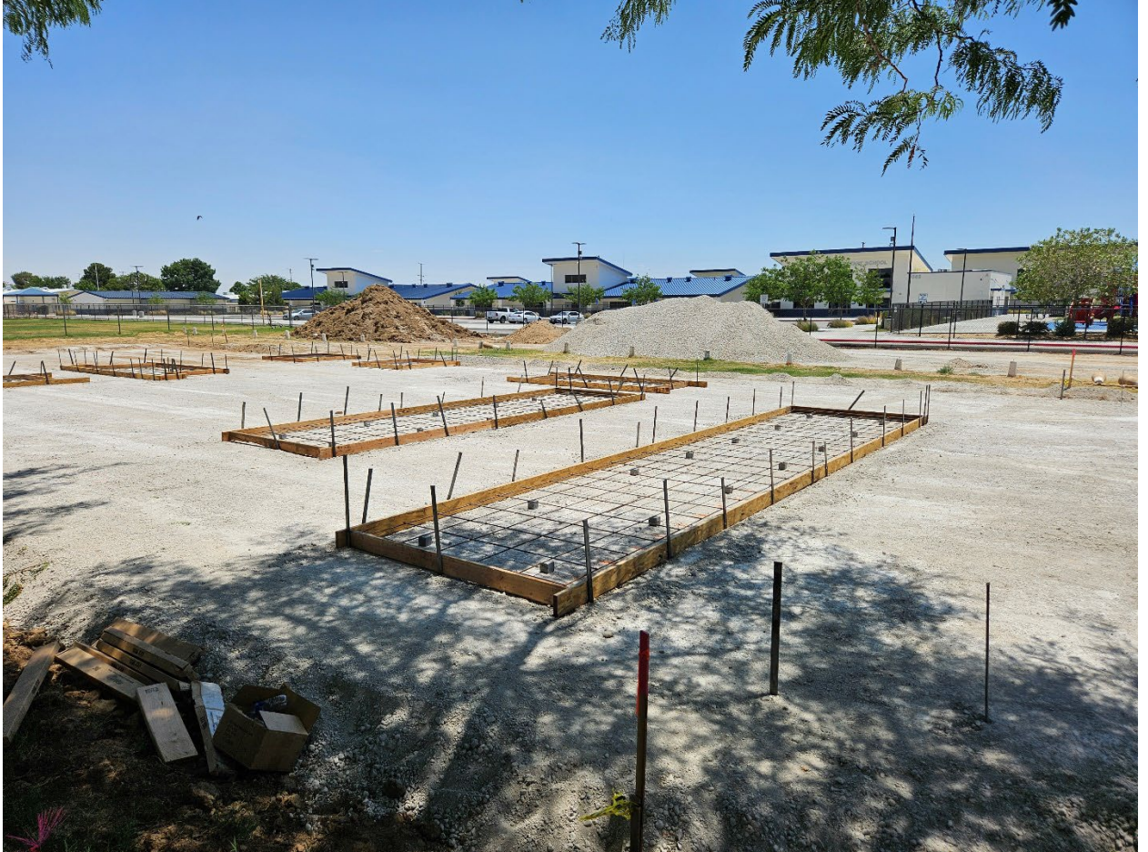
Skatepark under construction at Glendower Park
