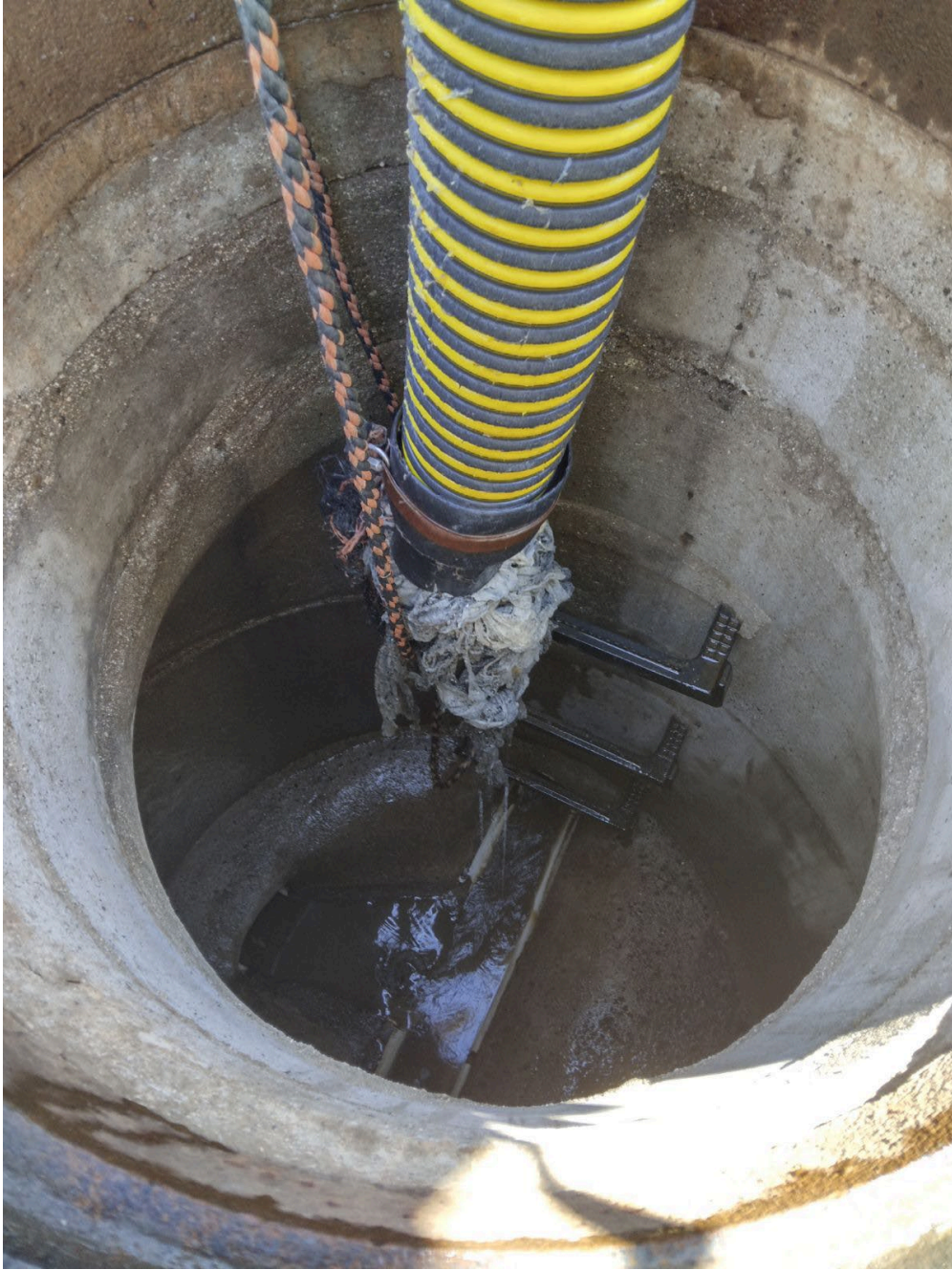
Debris and rag build up removed from sewer flow line
