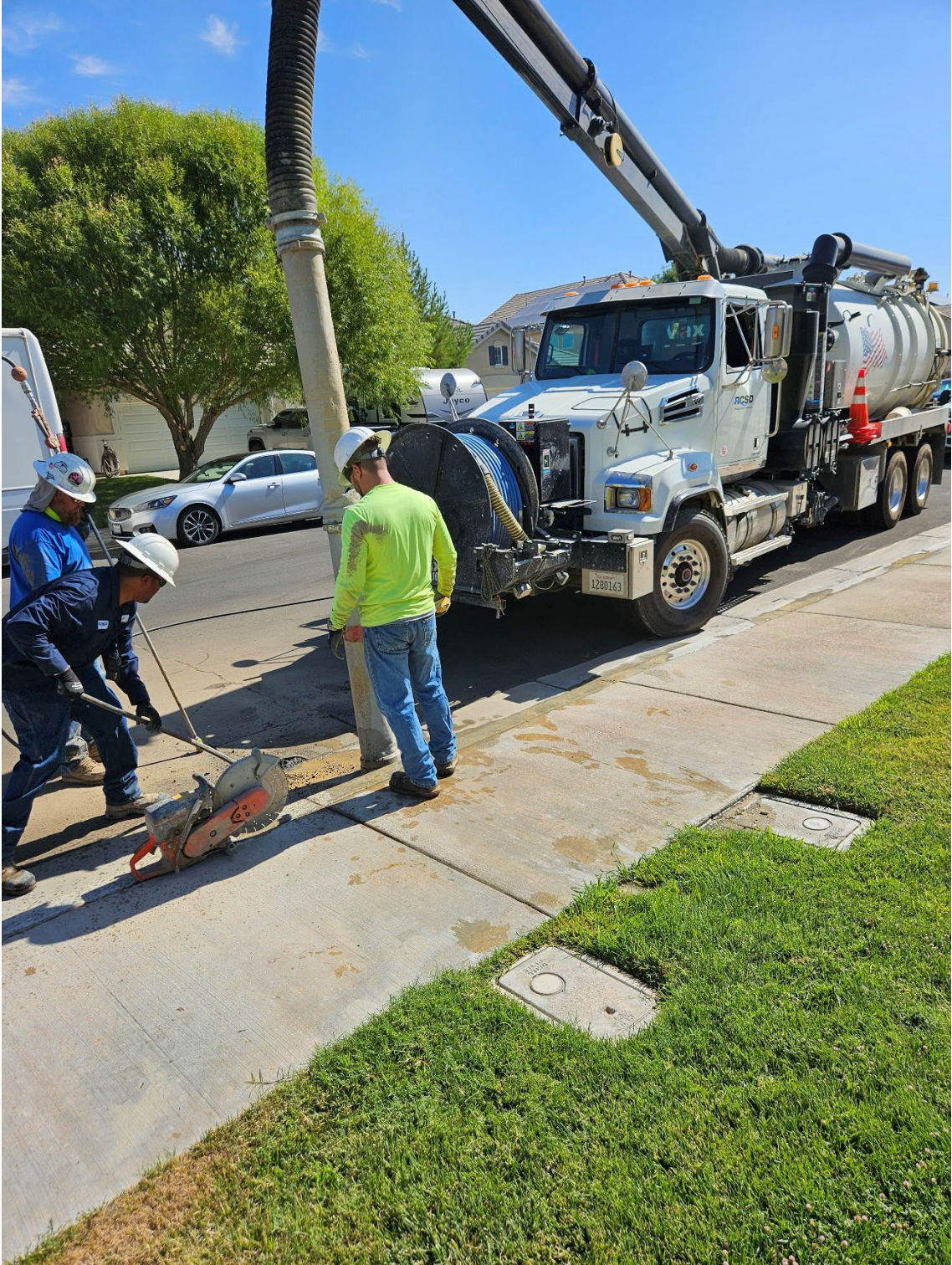
Public Works dept repairing water service line leak
