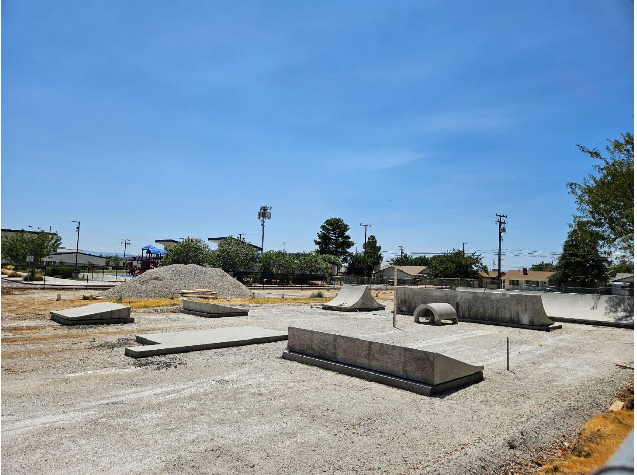
Construction of new concrete skatepark coming together
