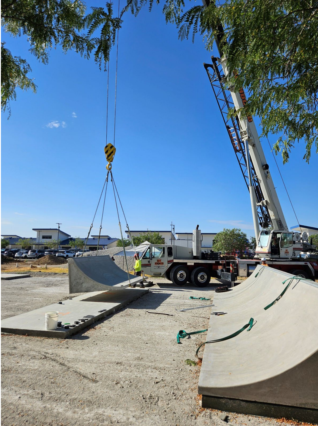
Concrete ramps being installed by crane.
