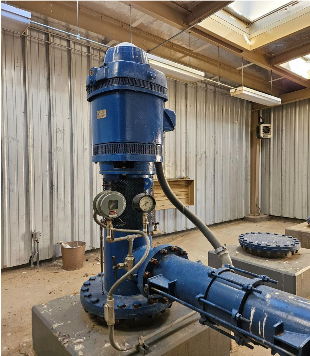
This is the booster pump that we had refurbished with new seals and shaft. This pump pushes water from tank 3 to tank 5.
