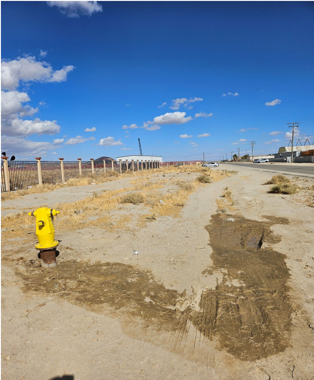
New Hydrant installation after thieves stole the existing hydrant.
