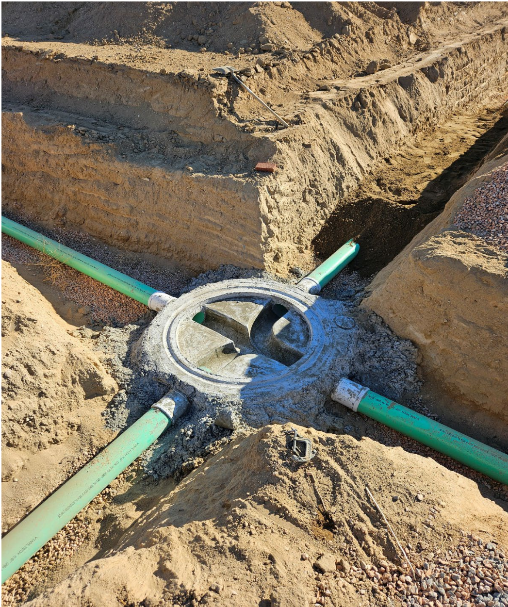
Finished concrete manhole shelf and channel and beginning to backfill.
