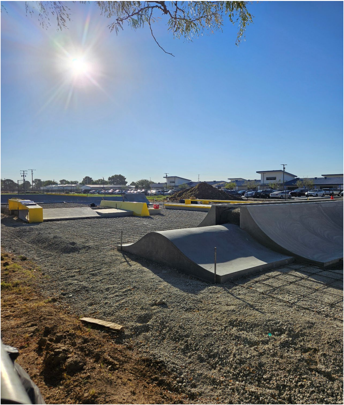
Skatepark nearing completion , expected to pour next week.
