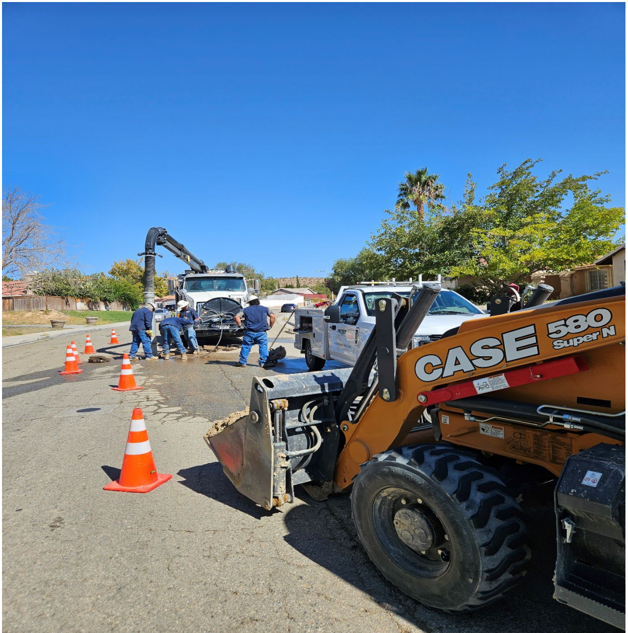
Public Works crew repairing a water line leak on Scherer st.
