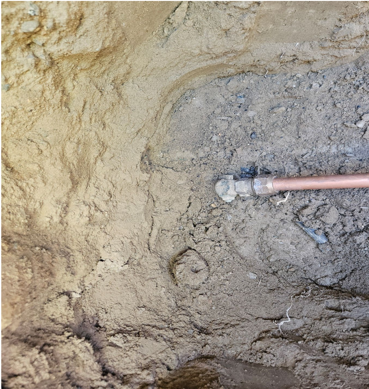
Copper services being installed by Lyles construction in the Trakell tract.
