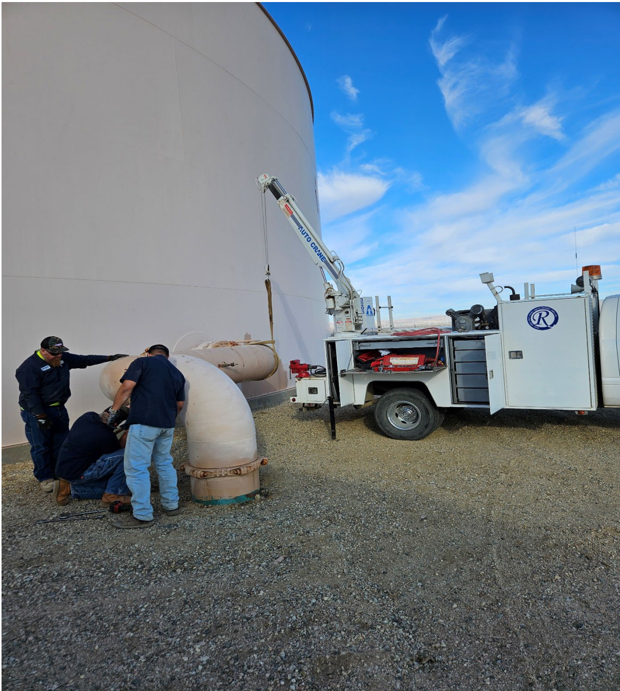
Victaulic coupling gaskets being repaired and replaced at Tank 5.
