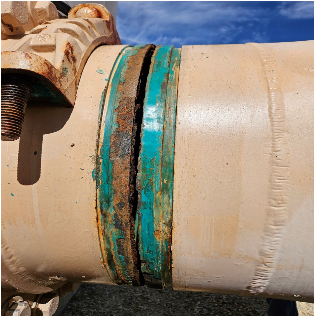
Inlet pipe at tank 5 before new gaskets were installed.
